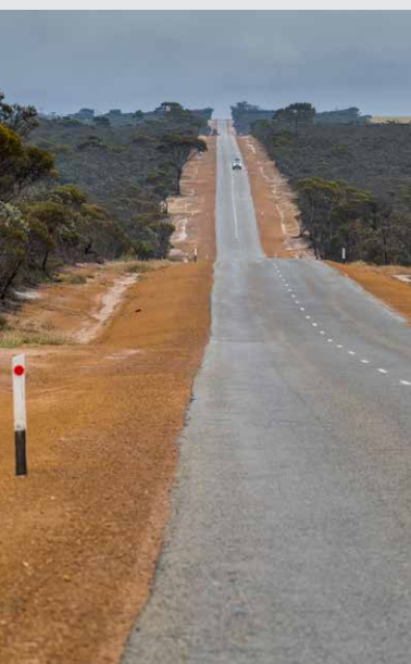
On major roads in Western Australia the average width managed from edge of the tar is 4m. AGRONOMO
