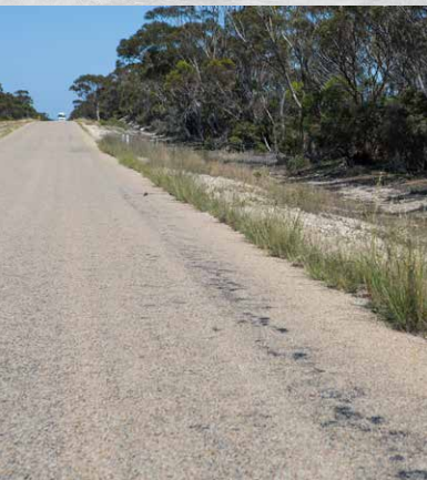
To maintain the integrity of the road base from ingress of water it is important to keep weeds from the edge of the tar. Perennial grasses are a problem because they are hard to control and thrive on the water harvested from the road surface. Grasspatch, WA. AGRONOMO
