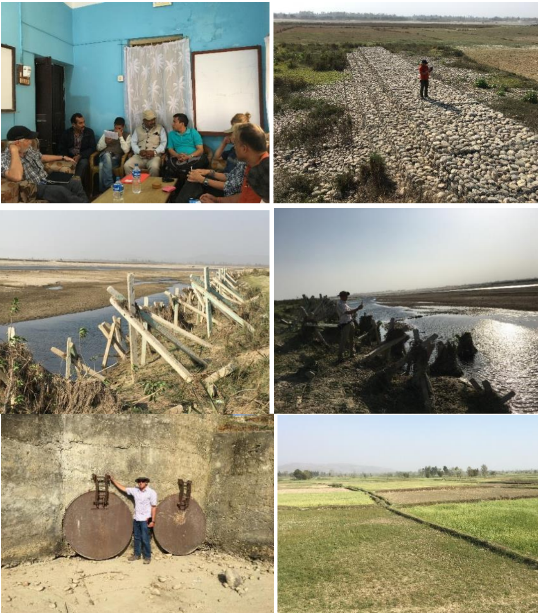
Figure 10 Meeting with engineer responsible for erosion control of the river bank; infrastructure (gabions) with rocks from the river (top right); concrete posts installed to reduce erosion of the riverbanks in Kamala River during the monsoon, the middle right shows the concrete post covered with sediments after two years of installation; infrastructure to divert water from flooded areas (bottom left) and irrigated paddock (bottom right)
