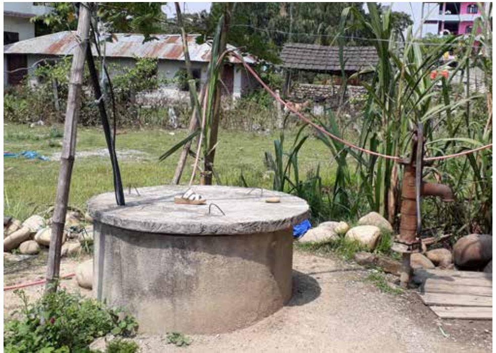
Figure 19 Open well and hand pump used for extracting water for domestic needs
