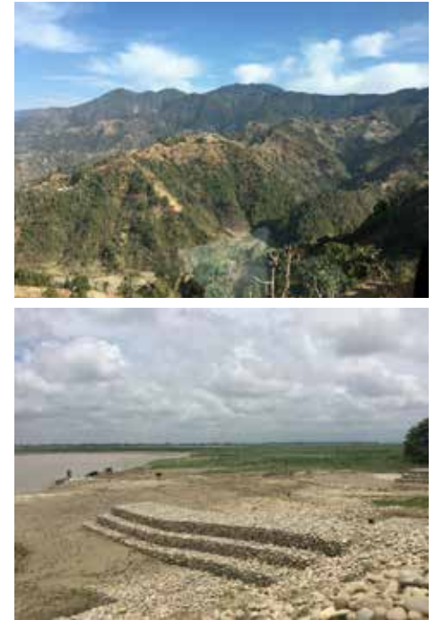
Figure 8 (Top) Unstable hills causing erosion and sedimentation Figure 9 (Bottom) Gabions built to protect the river banks
