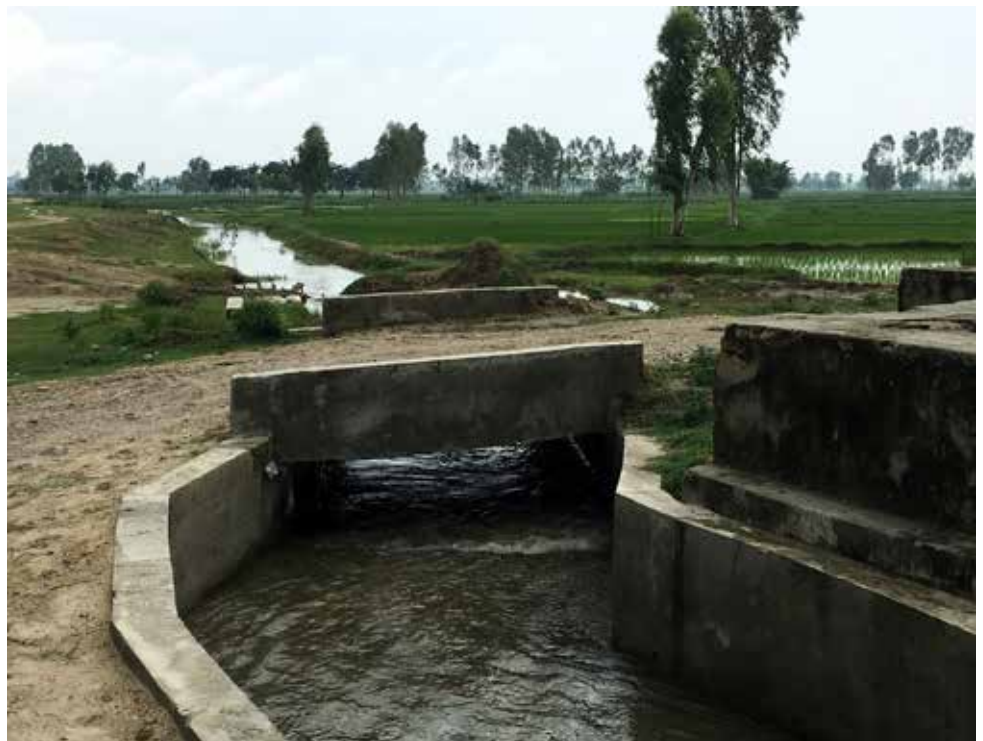
Figure 26 Kamala Irrigation Project command area (top) and irrigation canal branch (bottom)
