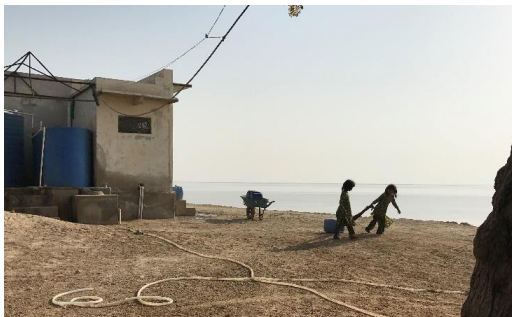
Girls collecting water from a reverse osmosis plant
