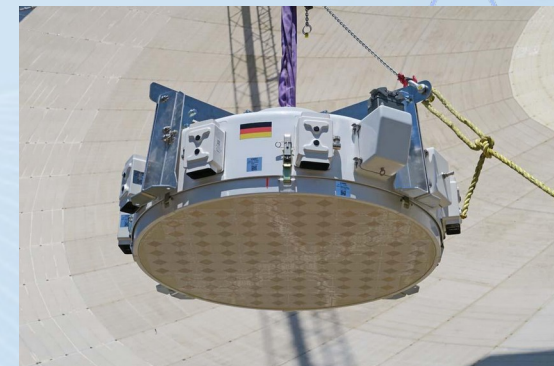
Top: CSIRO checkerboard PAF for the Effelsberg 100m telescope during its first installation (March 2017)
