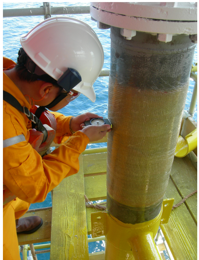
Badly deteriorated corrosion protection coating can be cost effectively replaced with PipeAssure™.
