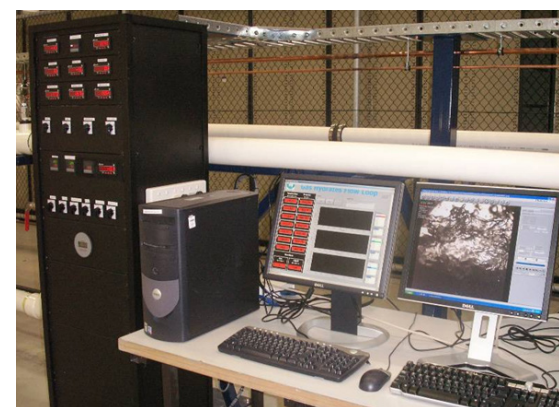
Data acquisition system.
