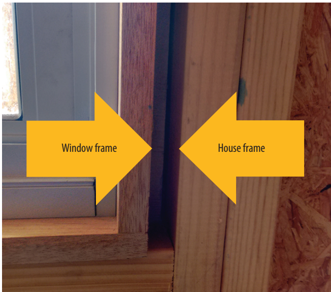
FIGURE 6 Unsealed gaps between windows and house frames let air pass through. (Michael Ambrose)
