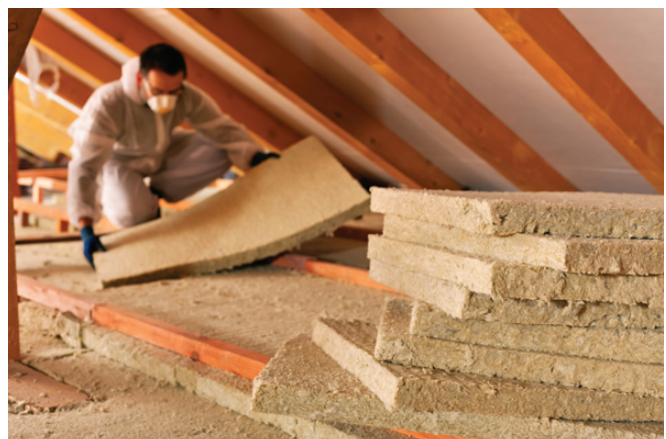
FIGURE 3 Protective equipment should be used when installing mineral fibre insulation. (Nagy-Bagoly Arpad/Shutterstock.com)
