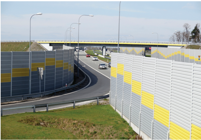
FIGURE 2 Noise-absorbing barriers (also called sound walls, noise walls, noise barriers, sound barriers or acoustical barriers) are often built next to motorways to manage traffic noise. (vladdon/Shutterstock)
