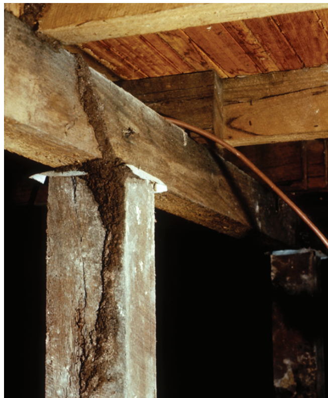
FIGURE 5 Termites reveal their presence by building a shelter tube to bypass an ant cap. (Forestry and Forest Products/CSIRO Science Image)
