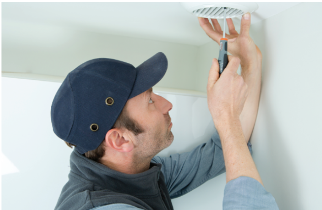
FIGURE 4 Air vents attached to the ceiling can remove moisture within a building. (ALPA PROD/Shutterstock)
