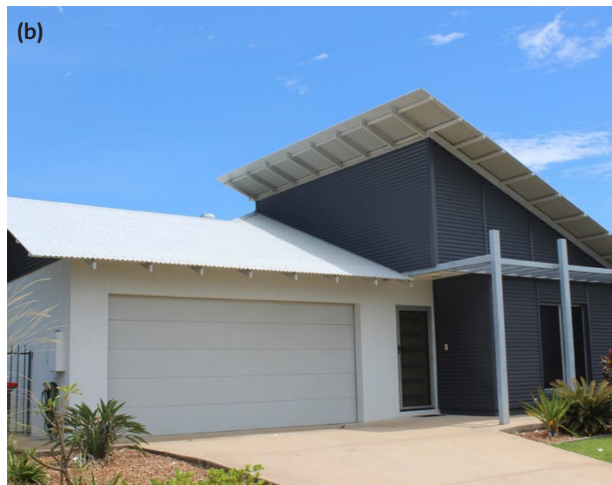
Figure 50. Darwin house design: (a) older design – elevated lightweight, (b) newer design – slab-on-ground heavyweight. Source: Williamson, T. (2023) Empirical validation of house rating software predictions and Darwinian’s thermal comfort thresholds, Darwin Home Comfort Rating Forum – March 2023.
