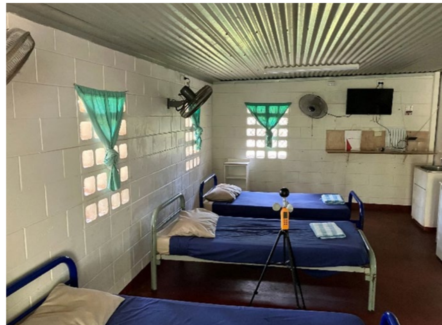
Figure 55. Two accommodation designs monitored in December 2023. Left: 'Village design', cement block walls of a light colour, uninsulated and unventilated roof with reflective foil (sarking), minimal shading by eaves with no eaves on the west and east orientations, ventilation provided by air bricks with little potential for cooling from cross breezes, and 450 mm mechanical wall-mounted fans. Right: 'Harmony design', cement block walls of a light colour, uninsulated and unventilated roof with reflective foil (sarking), rooms orientated to the north-west to capture prevailing breezes, large eaves providing shade, ventilation through louvre windows with 90% opening to the breeze, and ceiling fans.
