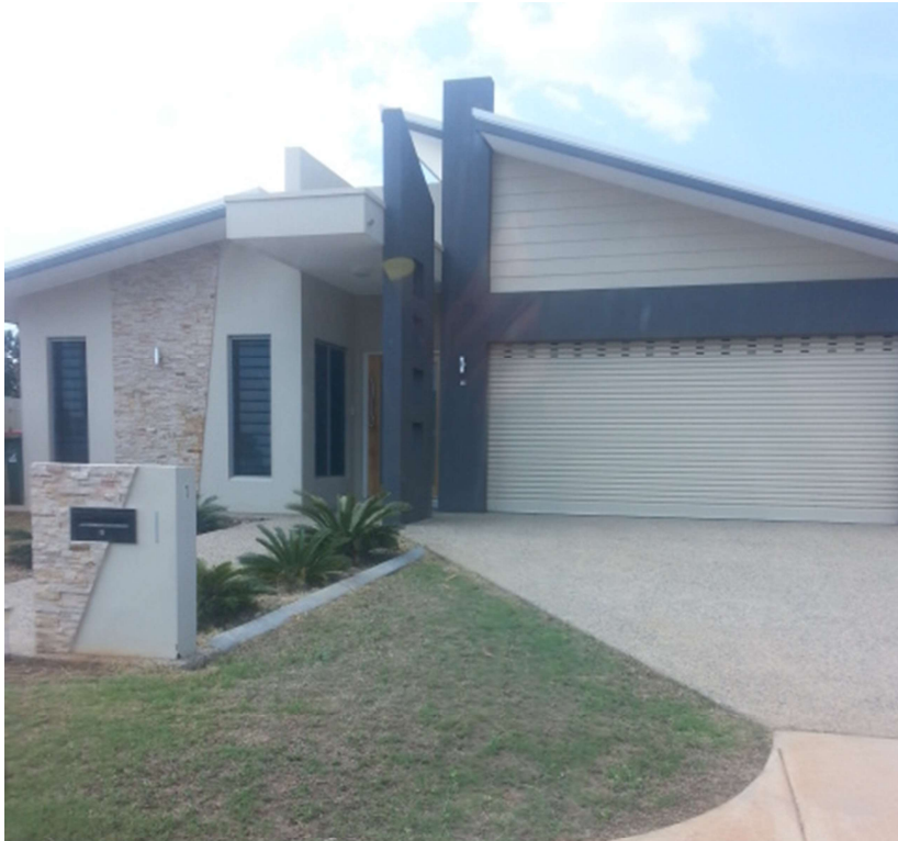
Single storey, concrete slab on ground, blockwork walls, colourbond roof
