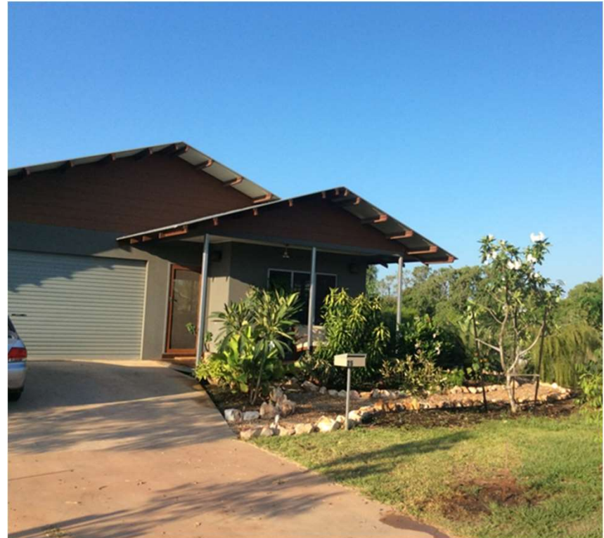
Single storey, concrete slab on-ground, fibro clad framed insulated walls
