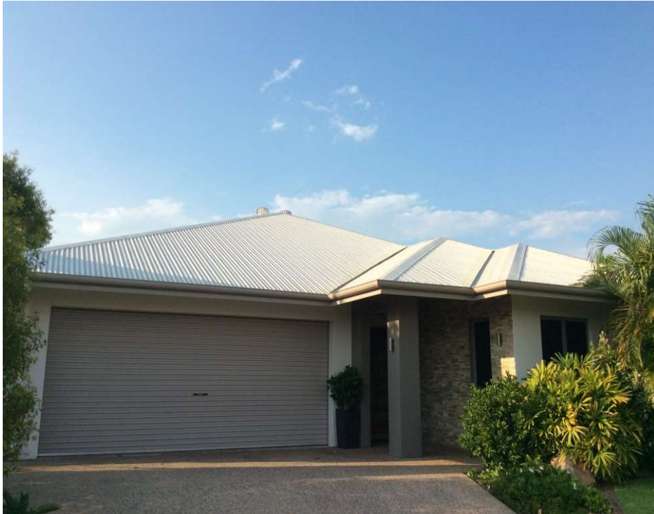
Single storey, concrete slab on ground, blockwork walls, colourbond roof
