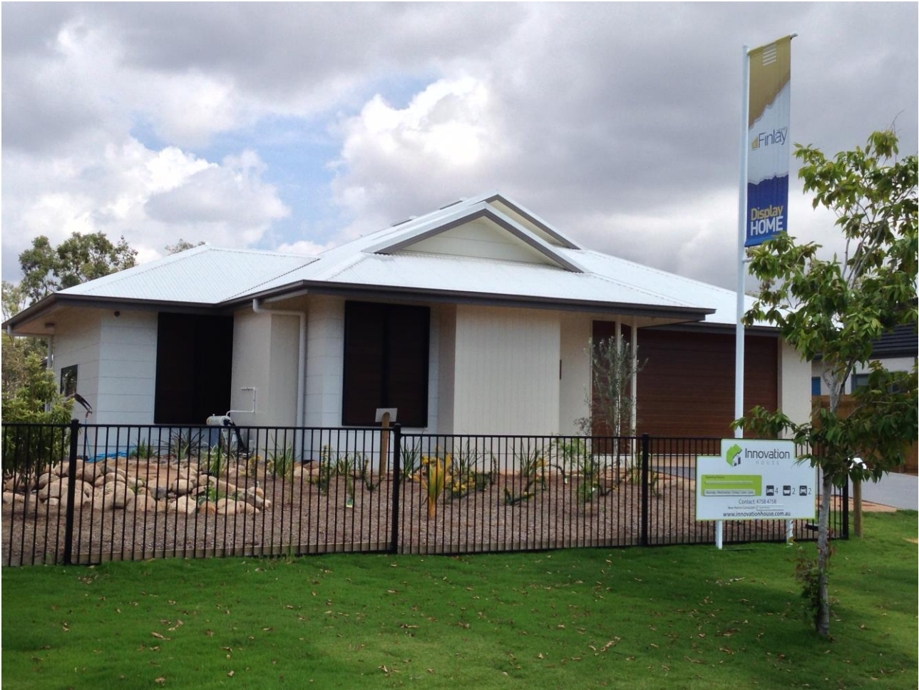
Image 3: Light coloured roof and walls reduce solar absorption (Supplied: Wendy Miller)
