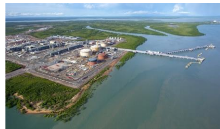
Construction of INPEX gas plant, Bladin Point near Darwin
