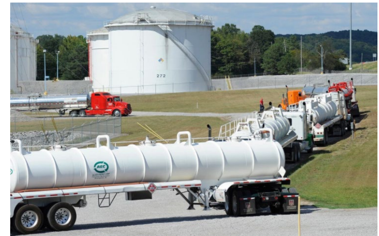
Colonial Pipeline (May 2021)
